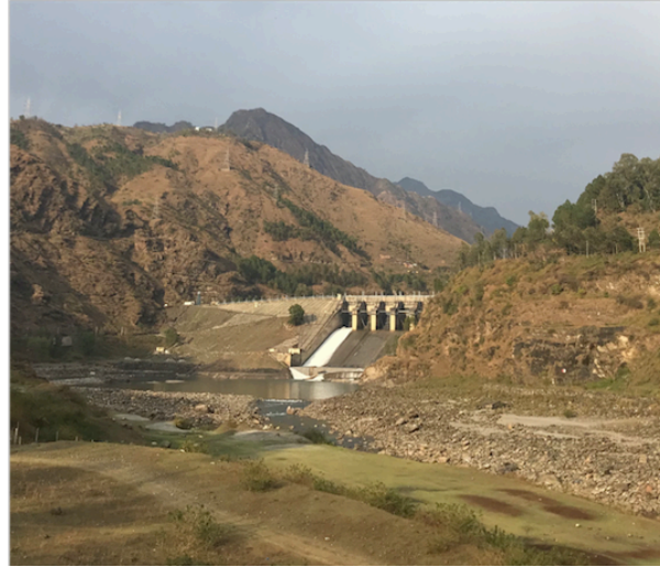
Figure 2.3: Pandoh Dam in Himachal Pradesh
