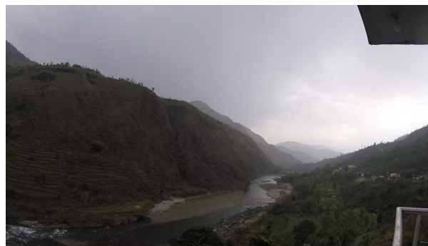
Figure 4.4: View of micro-turbine site
