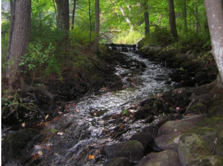
Figure 11 – Malden Brook flowing past spillway
