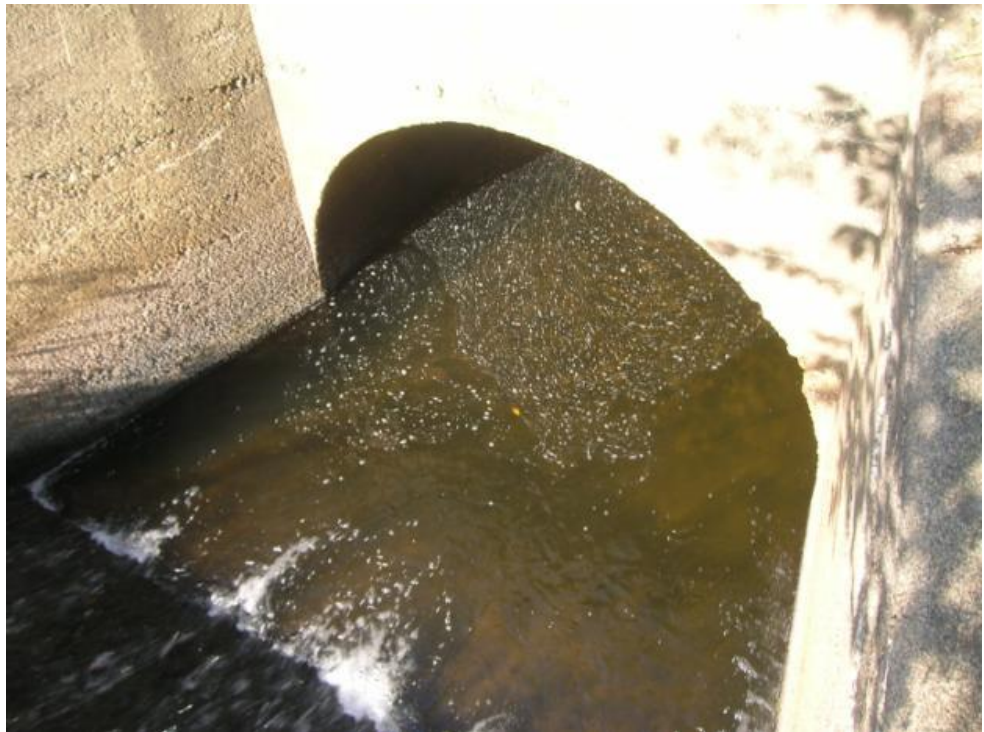
Figure 5 – Malden Brook culvert entering Wachusett Reservoir
