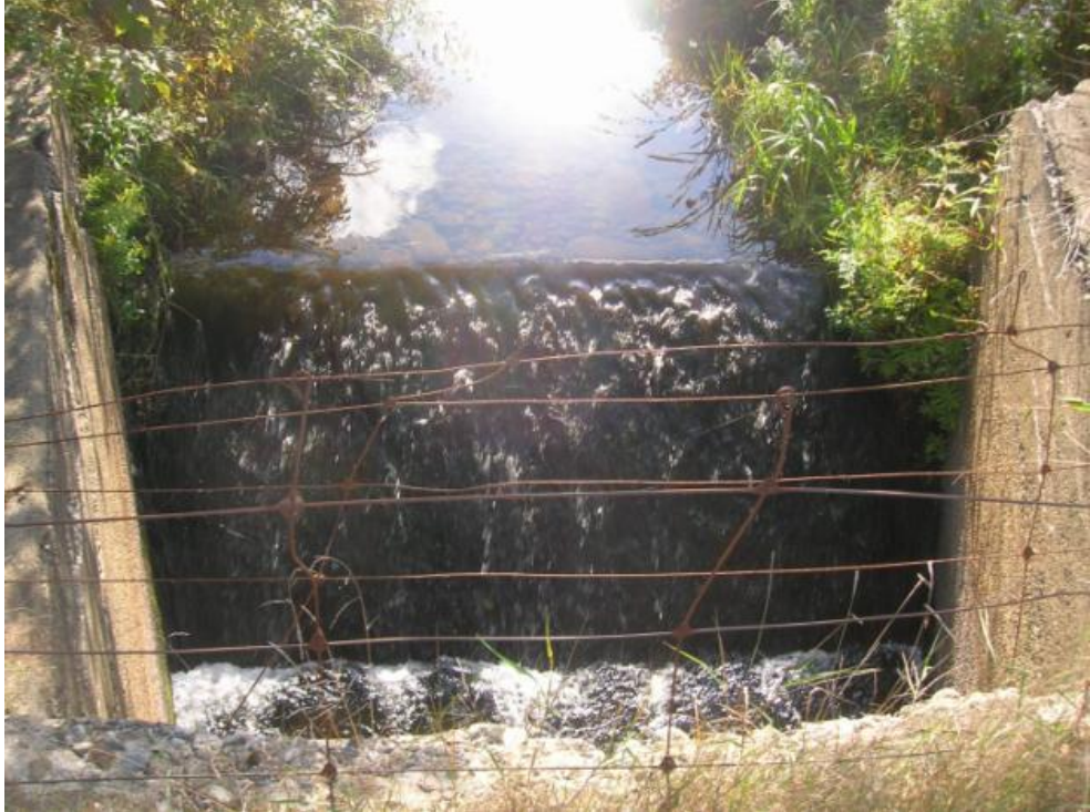
Figure 4 – Malden Brook culvert entering Wachusett Reservoir
