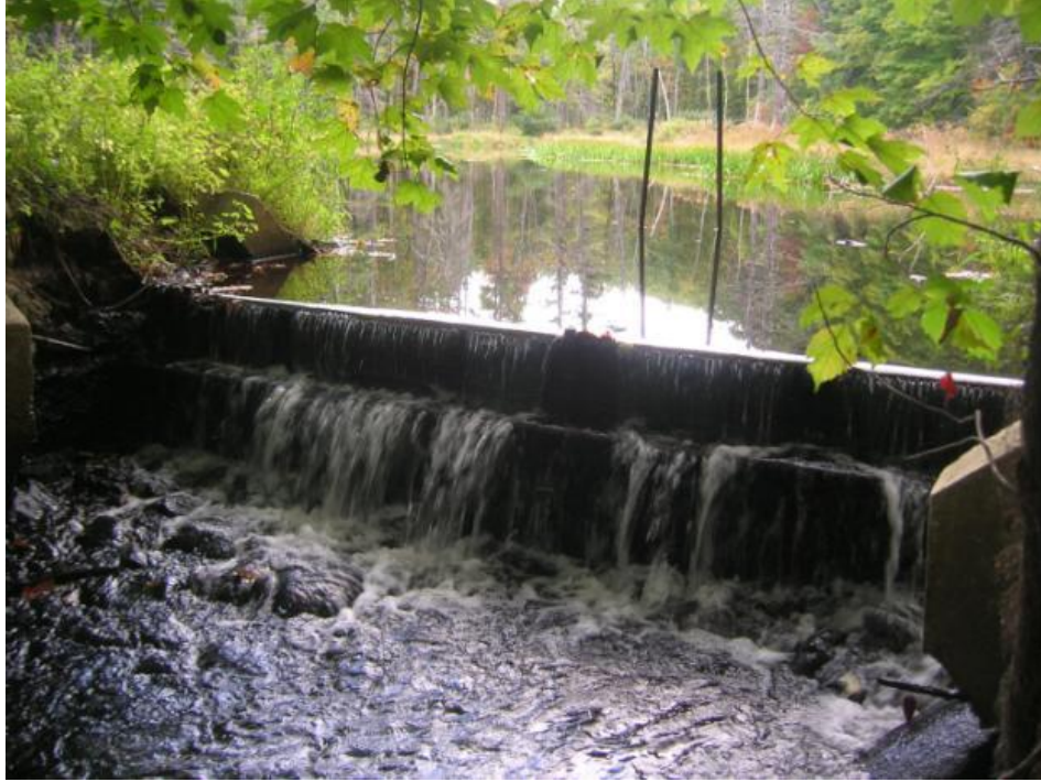
Figure 14 – Edwards Pond Dam spillway
