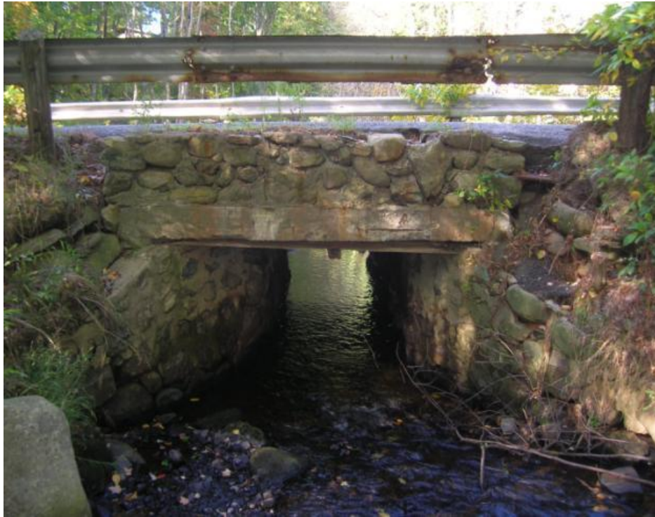
Figure 9 – Malden Brook Culvert view from upstream
