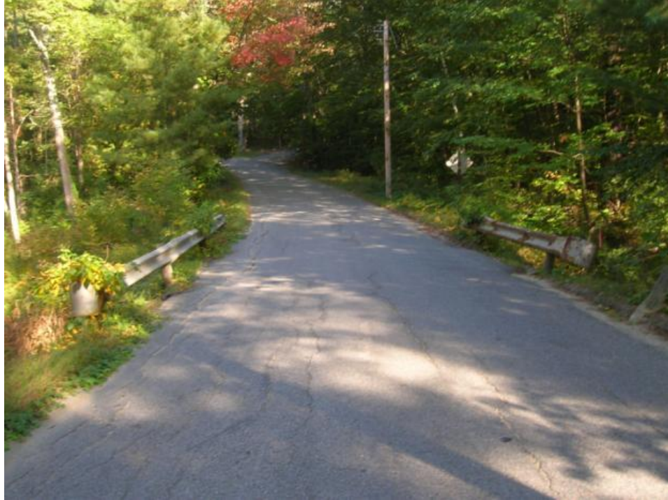
Figure 8 – Malden Street at Malden Brook Culvert
