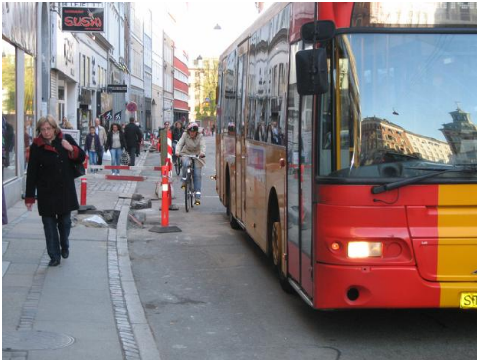
Figure 11: Busy Street with construction and no cycle path
