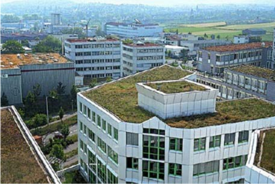
Figure 5- Extensive Green Roof
