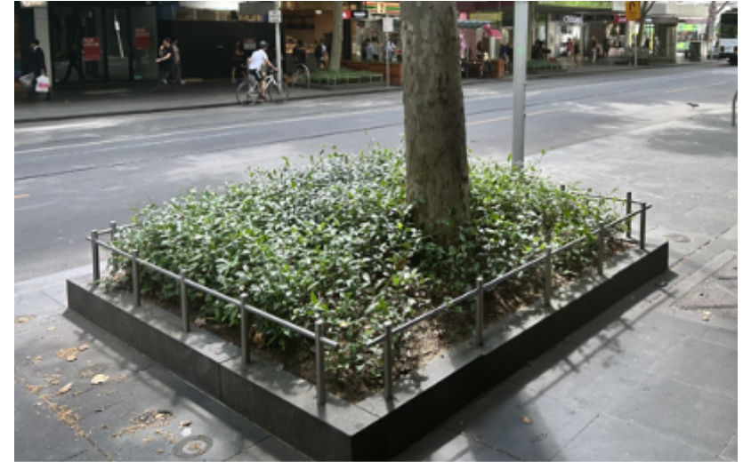
Figure 7: The image depicts a rain garden with a tree pit and demonstrates an example of blue infrastructure.
