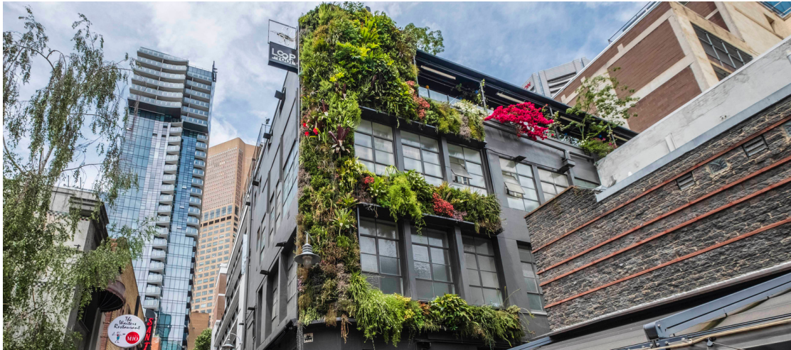
Figure 6: The image above demonstrates an example of green infrastructure around the city. This specific example is also referred to as a green wall. Photo credit to City of Melbourne.
