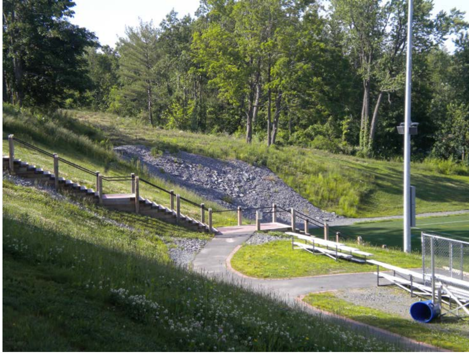
Slope and Stormwater Management at Multi-use Field at Becker College
