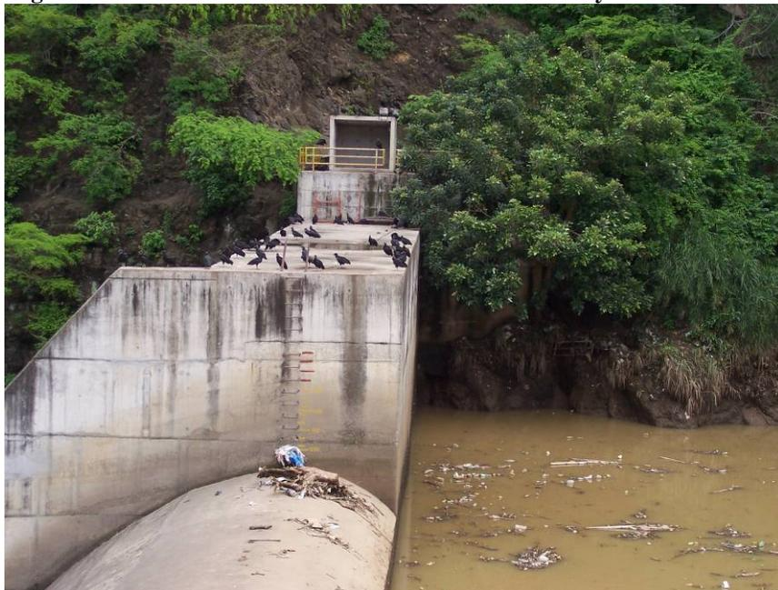
The dam is located at the junction of the Rio Uruca (from the Canton of Santa Ana) and the Rio Virilla (from the Cantons of Heredia and Moravia), with the hydropower works connected downstream by an 800 meter concrete canal (an underground tunnel) and a 600 meter long pipe. The pipe's diameter measures approximately 3 meters (Figure 4.3).
