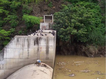
Figure 4.2: Dam and debris accumulation at the Brasil Hydroelectric Plant
