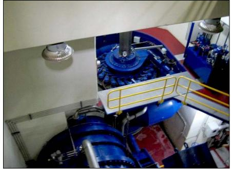
This system results in a 27 megawatt (maximum) facility. The water travels over a fall of 72 meters from the water intake at the dam to the turbine in the Brasil Plant. The turbine at the facility rotates at 300 revolutions per minute on a typical day, drawing 21 meters cubed per second of flow input and generating 14 megawatts of power (Figure 4.4). The maximum water flow is 34 meters cubed per second.
