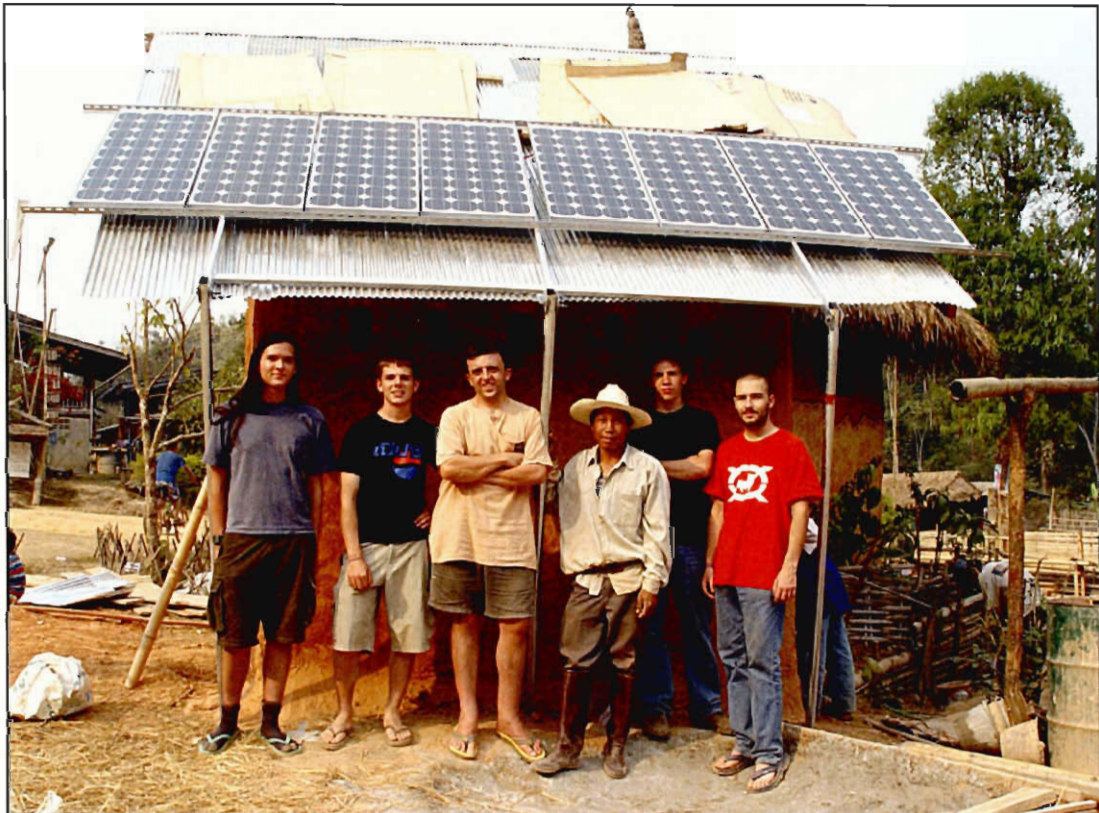
Figure 7: The completed solar module rack design
