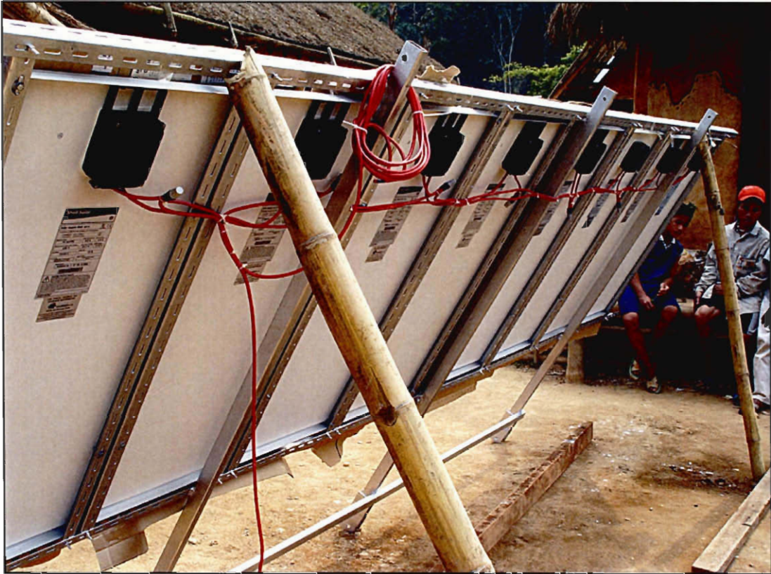
Figure 9: The solar array wired in parallel and series
