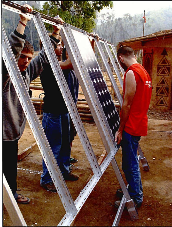
Figure 8: Bolting of solar panels into the frame
