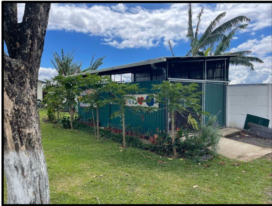
Figure 7: New Hope Collection Center Exterior.
