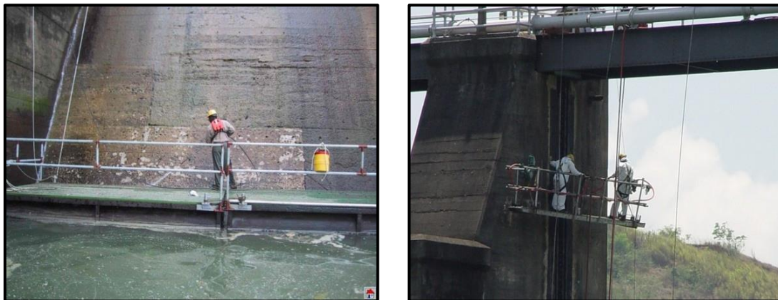
Figure 43: Existing floating (left) and mobile (right) scaffolding used by the ACP
