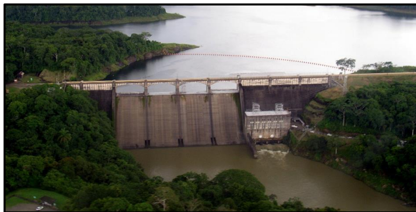
Figure 41: Madden Dam and Spillway with Alhajuela Lake in the background and the Chagres River in the foreground (justin_n, 2007)
