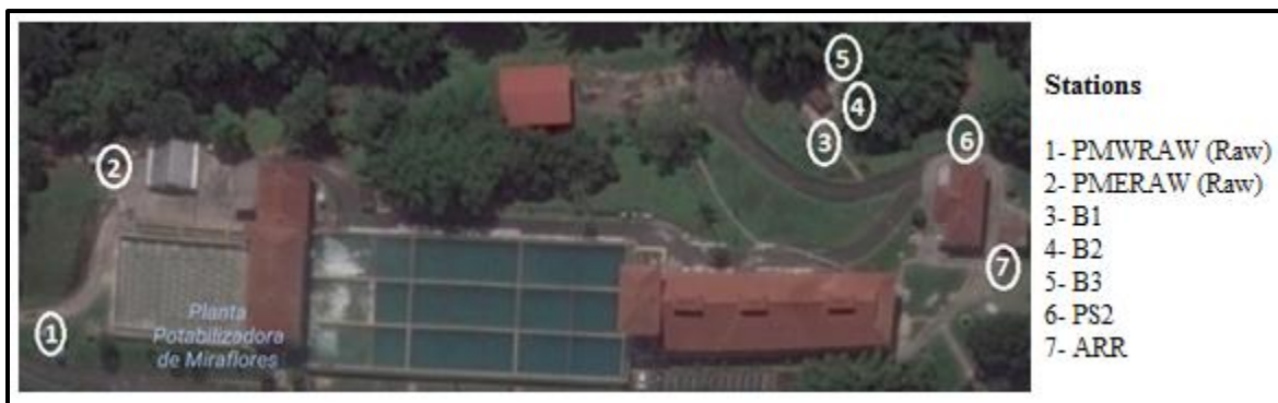
Figure 15: Water collection stations at Miraflores Water Treatment Plant (Google Maps, 2016)
