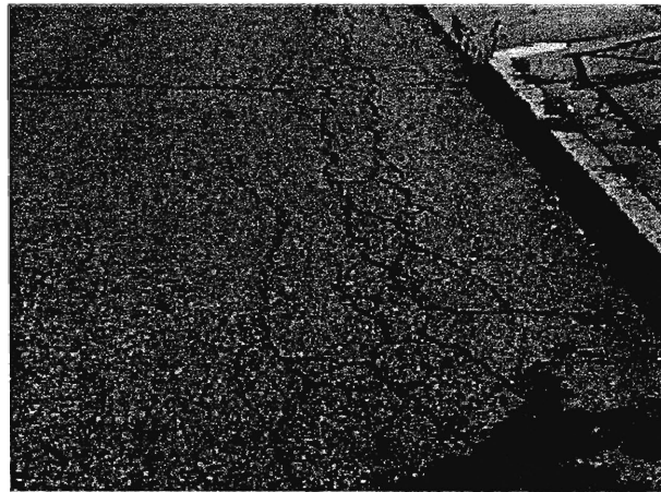
Figure 5. Cracking
