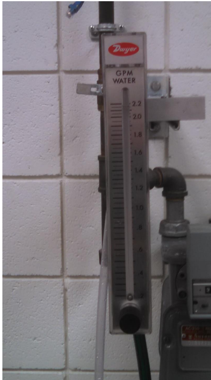
Figure 31: Rotameter in line with cold water tap.
