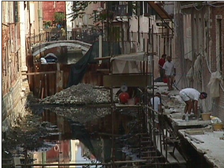
Figure 2: An example of the dry method of canal dredging
