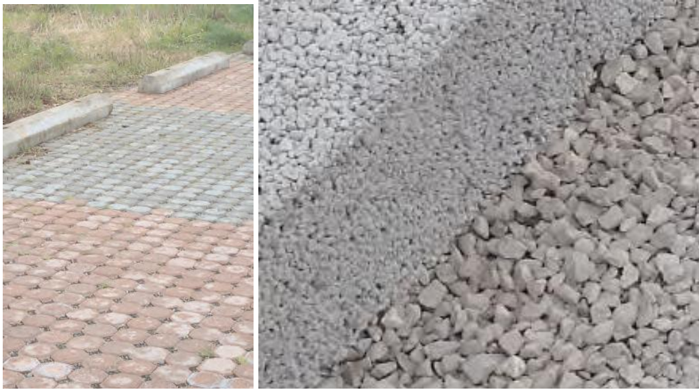
Figure 2-11: Pervious pavement (Environmental Services City of Portland, 2006)
