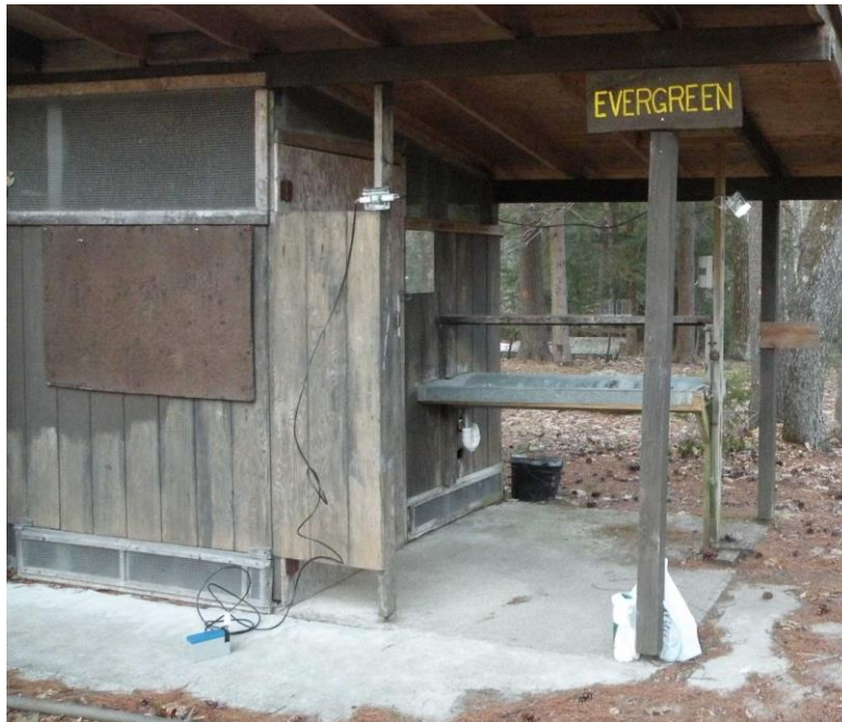
Figure 43: Sensor and light installation at latrine
