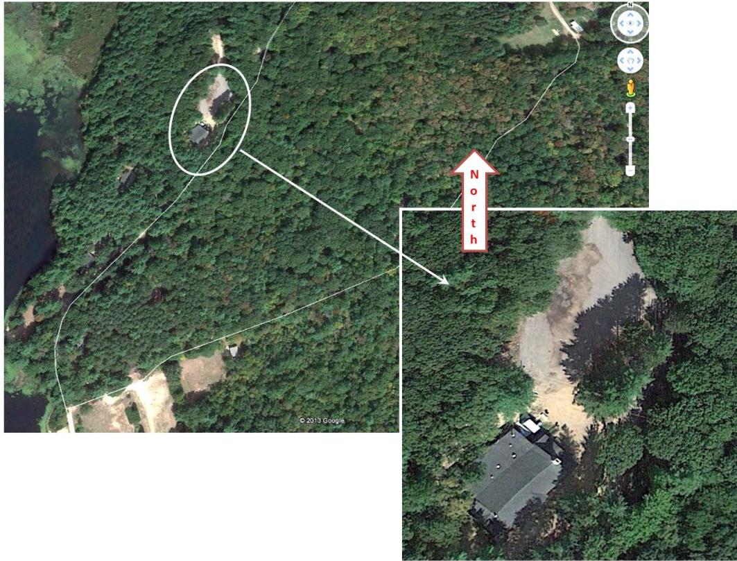
Figure 12: Aerial view of East Lodge solar site
