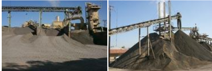
Stockpile and Conveyor System
