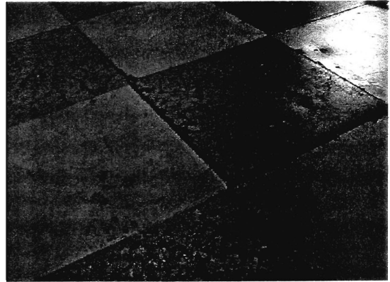
Figure 28: An example of a joint gap
