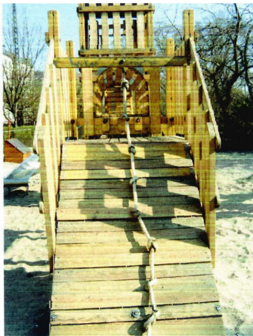
Fig. 4.25: Protective Railings and Handrails
