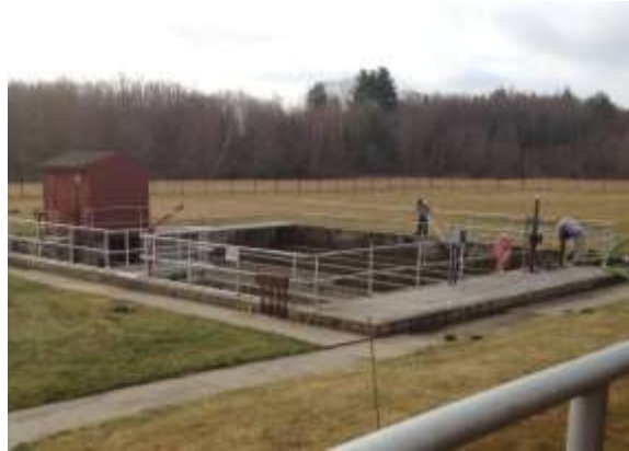
Figure 12: Chlorine contact tank for disinfection
