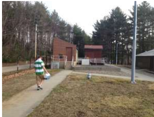
Figure 8: Gardner WWTF headworks building
