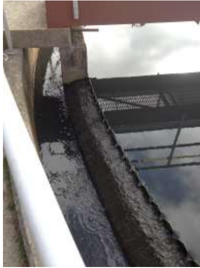
Figure 21: Location of intermediate clarifier sampling
