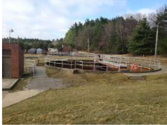
Figure 9: Gardner WWTF primary clarifiers
