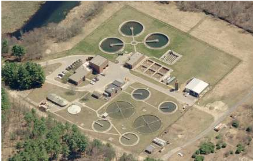
Figure 5: Aerial View of the Gardner WWTF
