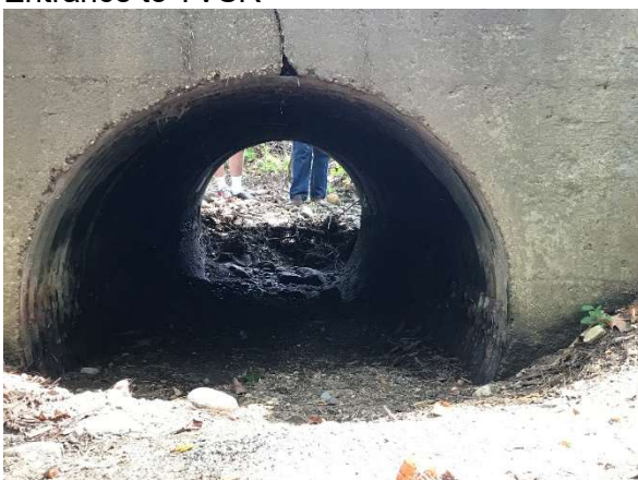
Existing Culvert under Snake River Road
