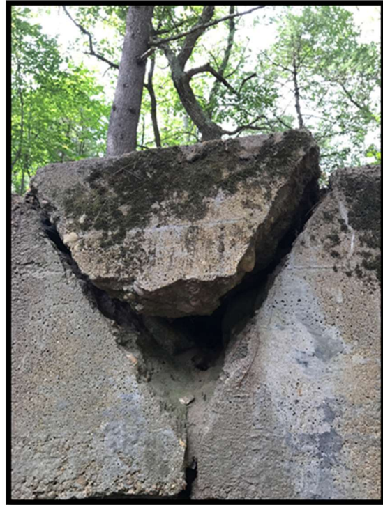
Figure 14 (Left): Substantial Wear on Concrete Bridge 1
