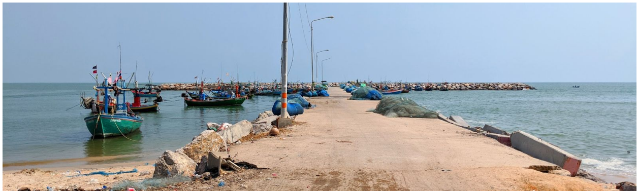
Figure 3: Photo of Groyne Meeting a Breakwater in Front of the Bang Kwai Community
