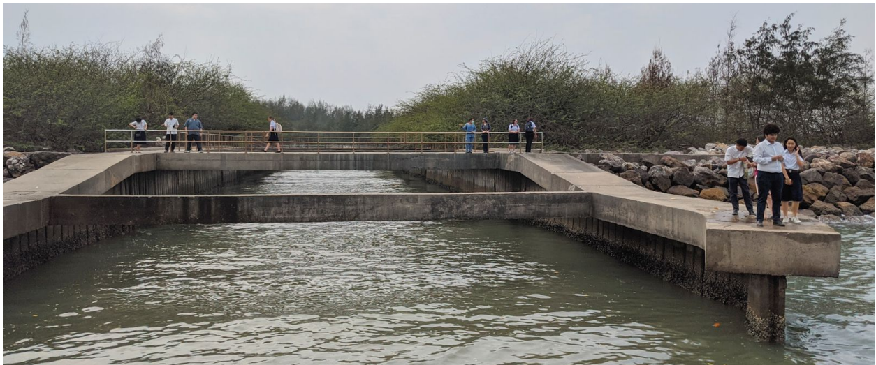
Figure 2: Photo of North Jetty
