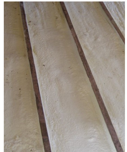
Spray foam insulation in the attic floor boards
