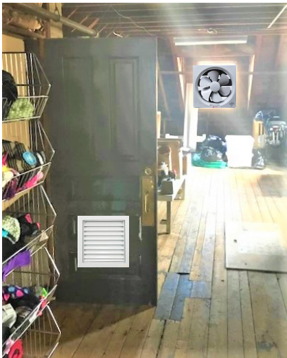
Adding in an exhaust fan and door grille to the attic
