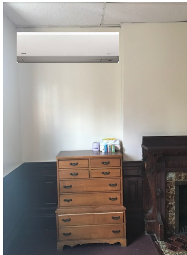
Adding heat pumps in the residents room
