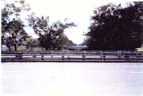
View South from J.T. Pinero Avenue
