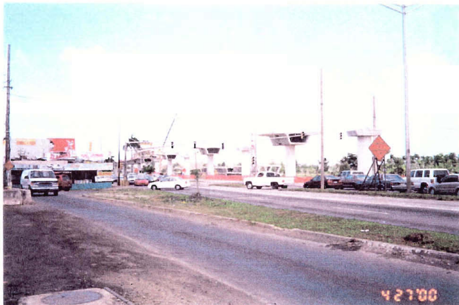
Figure 4.20 Tren Urbano Construction
