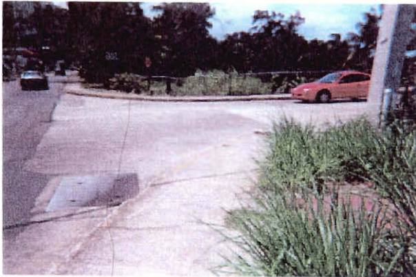
View North of Roadway Crossing Notra Dame Bridge
