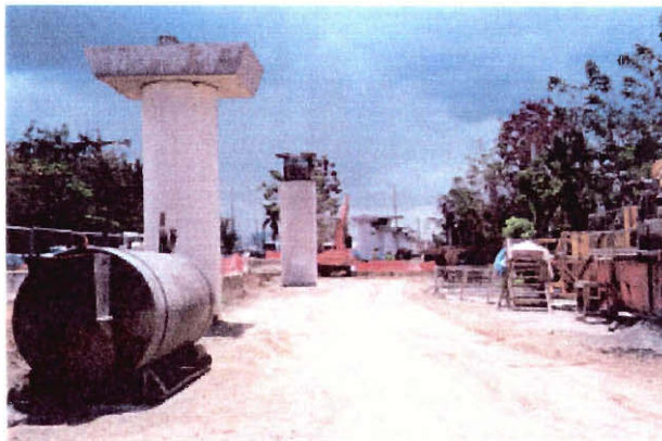
Tren Urbano Construction Parallel to PRI
