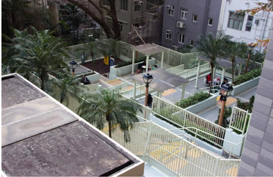
Figure 4.7 Kwon Hon Terrace Garden, Note: Number of fences and number of people
