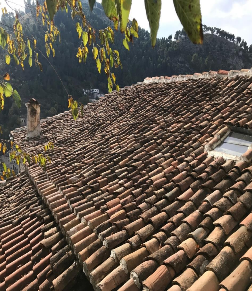
Figure 35 Historical Content: Roof
