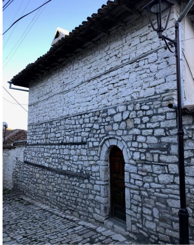
Figure 36 Historical Content: Outer Walls
