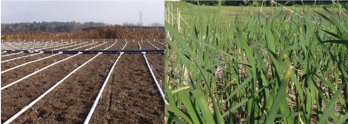
Figure 30: Finished VF Wetland Before and After Plants Have Grown (AQUA Treatment Technologies, 2008)
