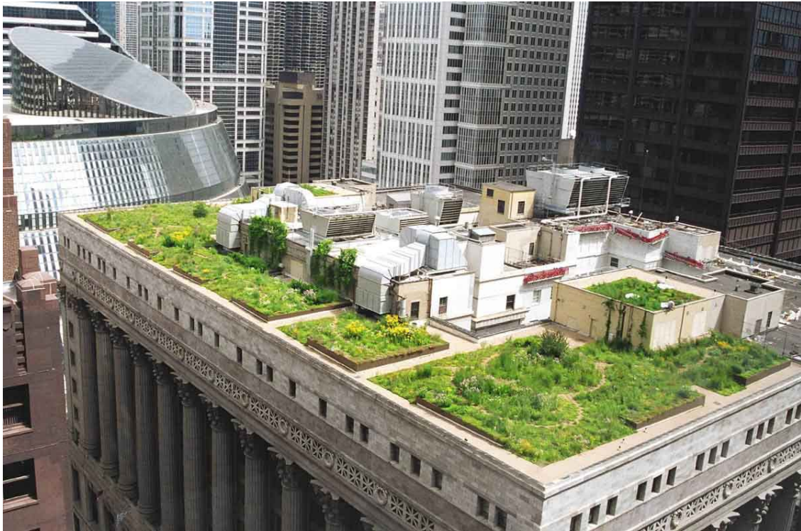
Figure 8: Extensive Green Roof on Chicago City Hall
