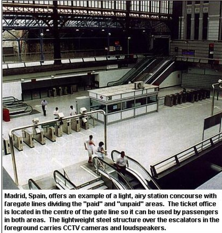
Figure 3, Concourse Design: The photo was taken in Madrid, Spain. It offers an example of a light, airy station concourse with fare gate lines dividing the "paid" and "unpaid" areas. The ticket office is located at the center of the gate line so it can be used by passengers in both areas. The lightweight steel structure over the escalators (bottom left of photo) allows CCTV (Closed Circuit Television) cameras and loudspeakers to be hung.
