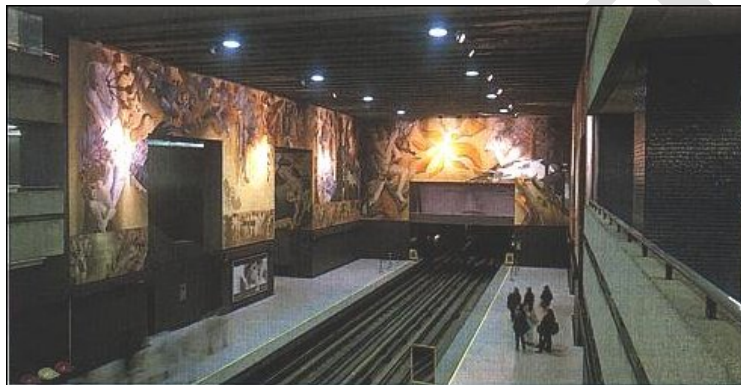
A new underground station on the metro system of Santiago, Chile. A combination of striking architecture and subdued lighting combine to give a pleasing overall finish. The use of upper level galleries, visible to the left and right, is unusual but adds to the feeling of accessibility.
