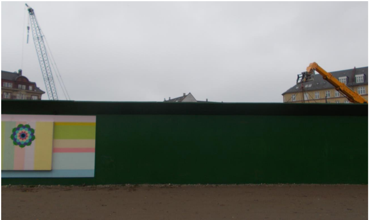
Figure 6.1.g: Faelledparken, location E, construction site barrier close up
