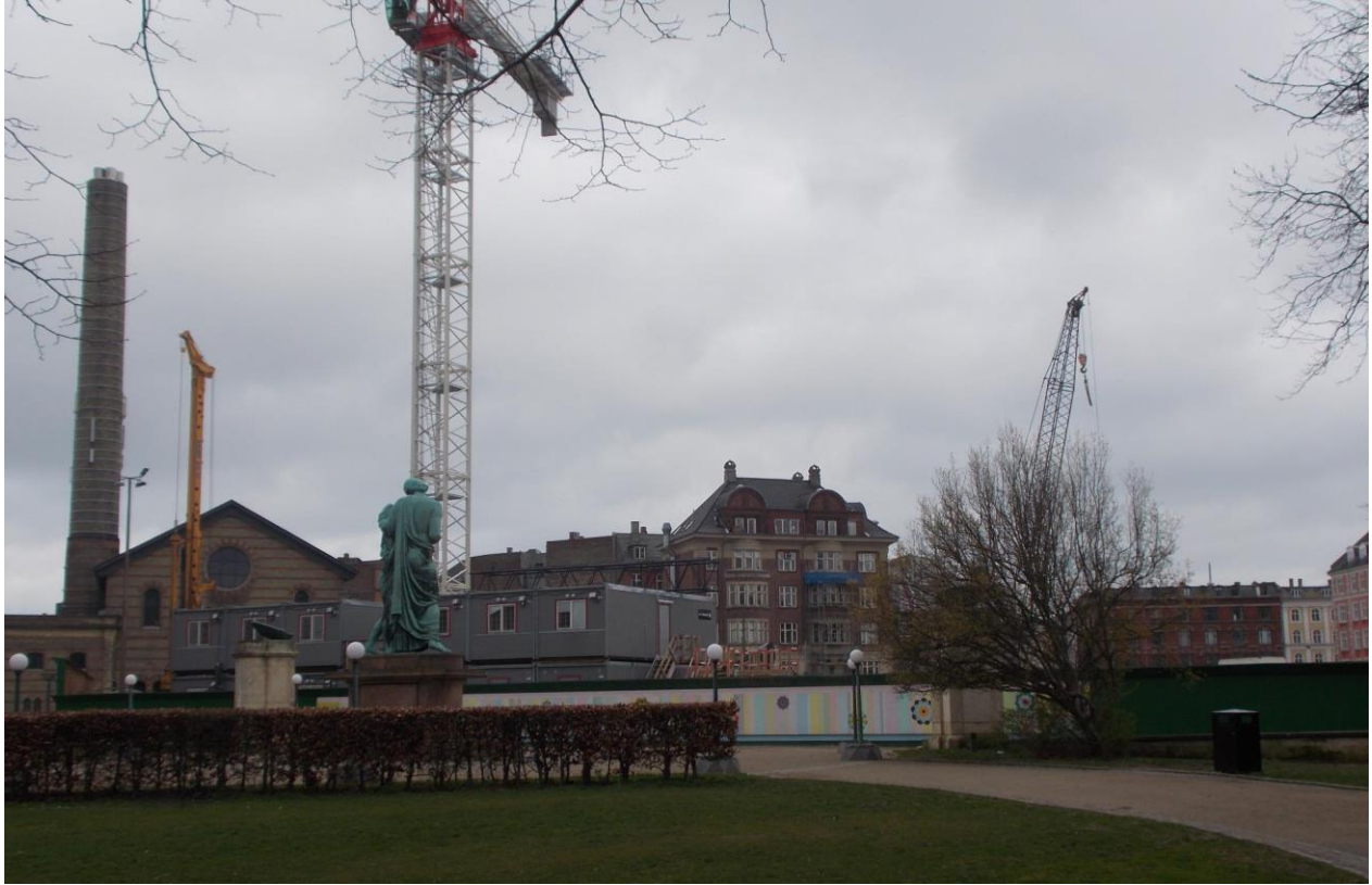
Figure 7.1.p: Faelledparken Construction Site Barriers
