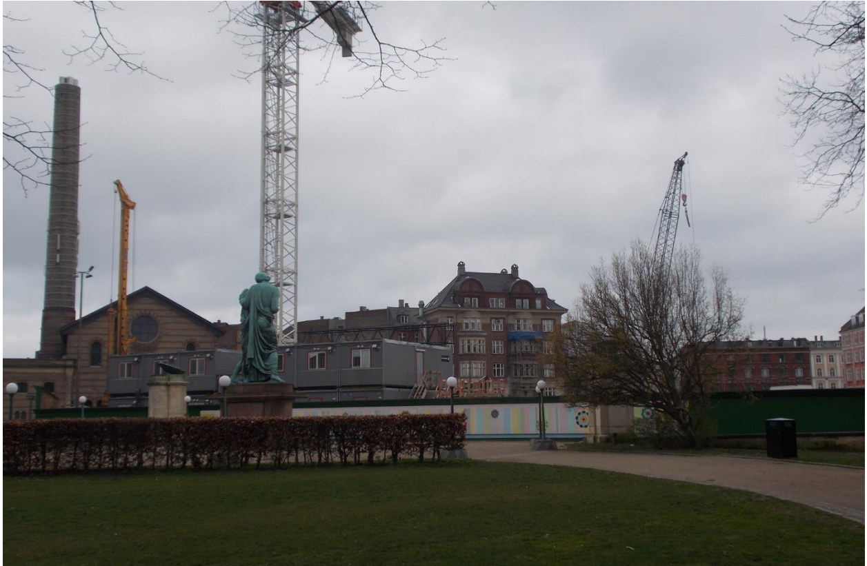
Figure 6.1.f: Faelledparken, location E, construction site with barriers
