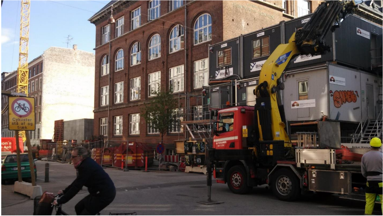
Figure 6.1.c: Langelinieskolen with visible, active construction next to school
