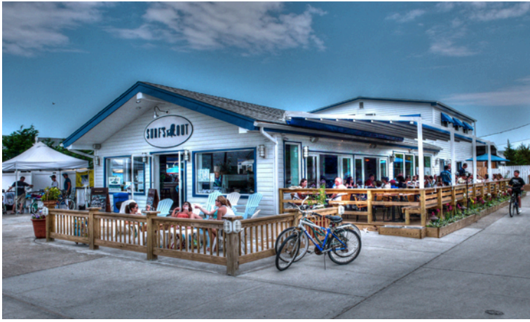
Figure 23 Surfs & Out Restaurant, Fire Island, Long Island, New York
