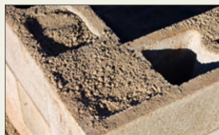
Figure 14. Reinforcing the Cinderblocks with Concrete Mix. Source: http://wildgingerfarm.com/ConcreteBlockRaisedBed.htm
