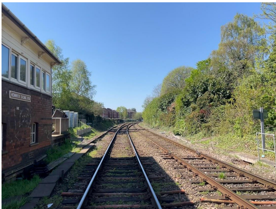
Figure 13: The remaining signal Box at Henwick Station. (Stone, 2023)
