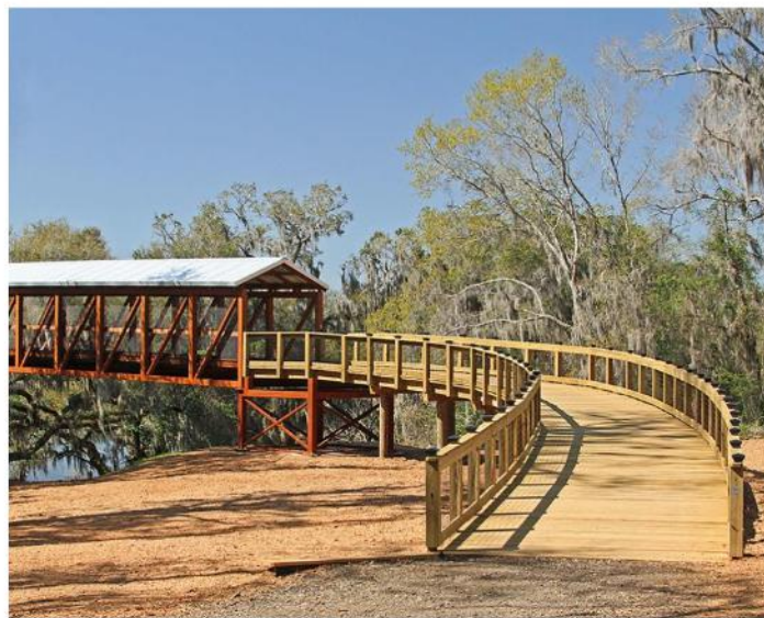
Figure 9: Wooden pedestrian bridge at Lafayette Heritage Park (Pedestrian, 2015)
