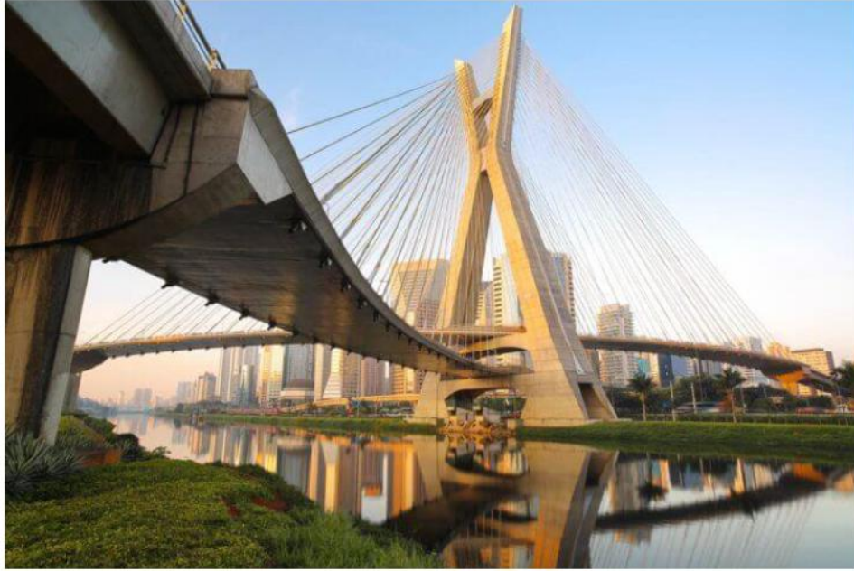
Figure 8: Picture of Octavio Frias de Oliveira bridge (Octavio)
