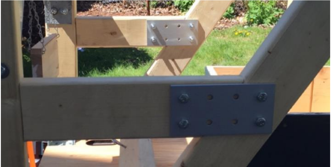
Figure 66 Wood Angle Beams
