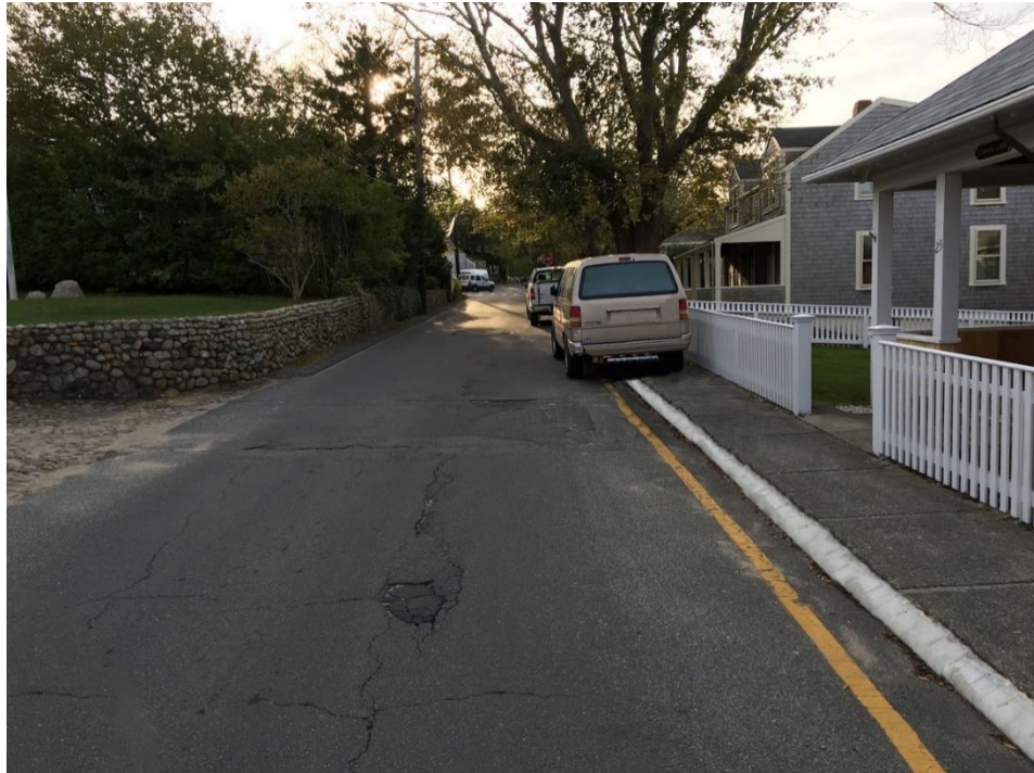
Figure 28: York Street with Mountable Curb
