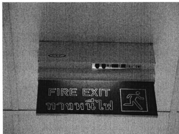
Figure 8: Fire Exit Sign
