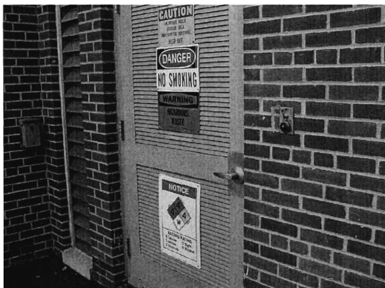
Figure 28- Entrance to MAA, with warnings and placards
