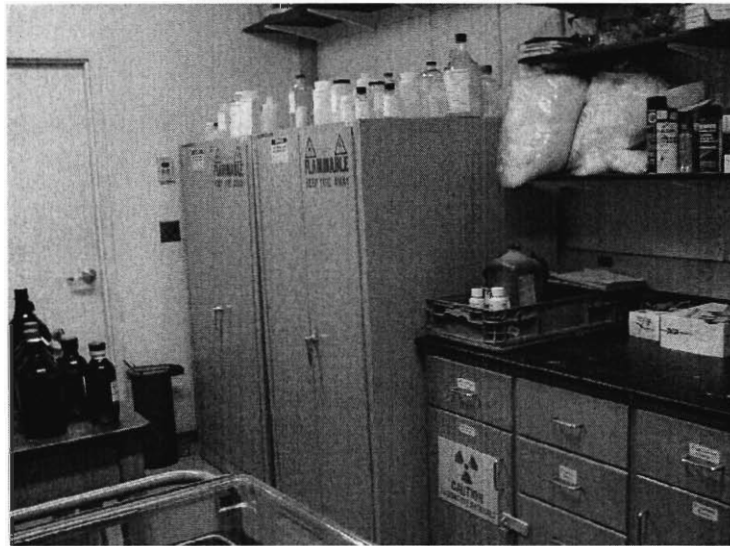
Figure 34 - Flammable materials cabinet
