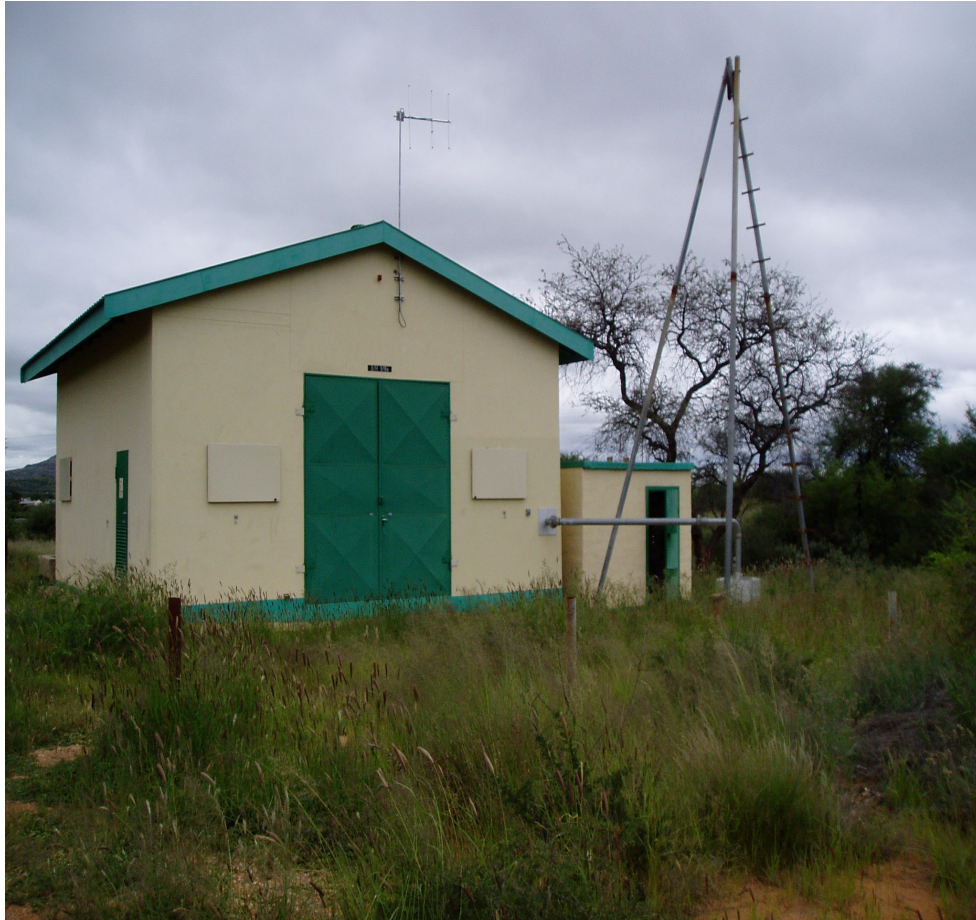
Figure 2 -Borehole Station in Windhoek
