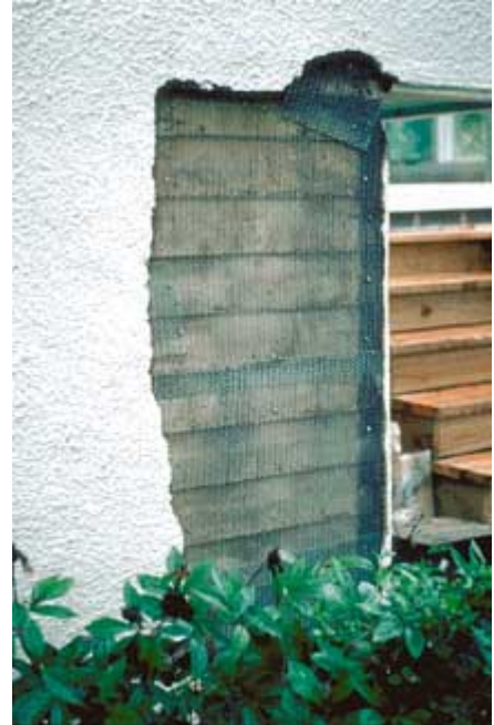
Preparation for stucco repair.
