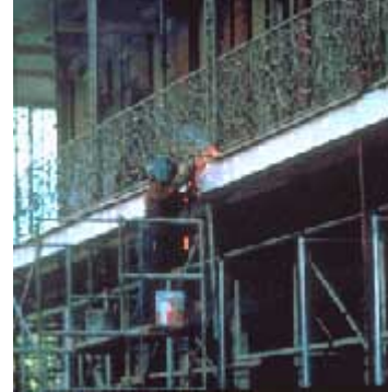
Repairing a decorative iron balcony.
