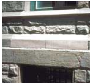
Replacement stones tooled to match original.
