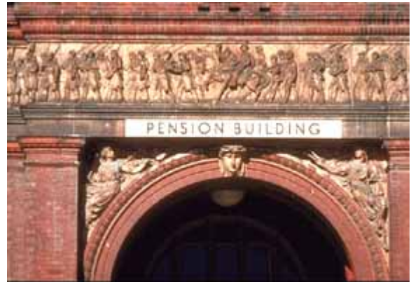
1880s brick building with terra-cotta trim.
