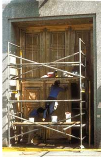
Applying a protective coating to bronze doors after cleaning.
