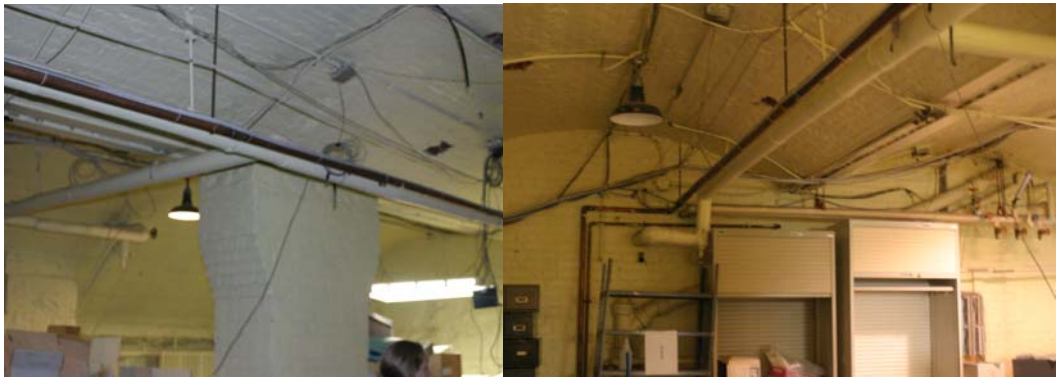
Figure 2: Photos showing segmented arch and brick pilaster
