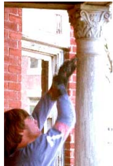
Hand scraping wood column prior to repainting.
