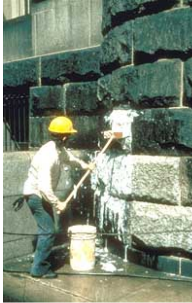
Chemical cleaning to remove dirt from granite.
