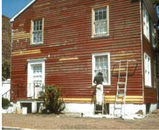
Limited replacement-in-kind of deteriorated wood clapboards.
