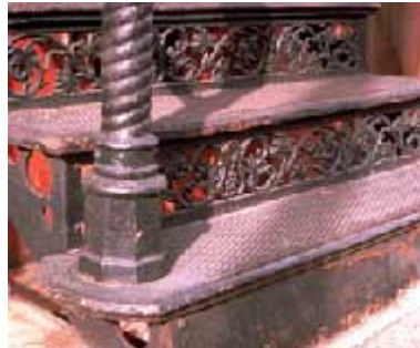
Cast-iron steps with distinctive cut-out work.
