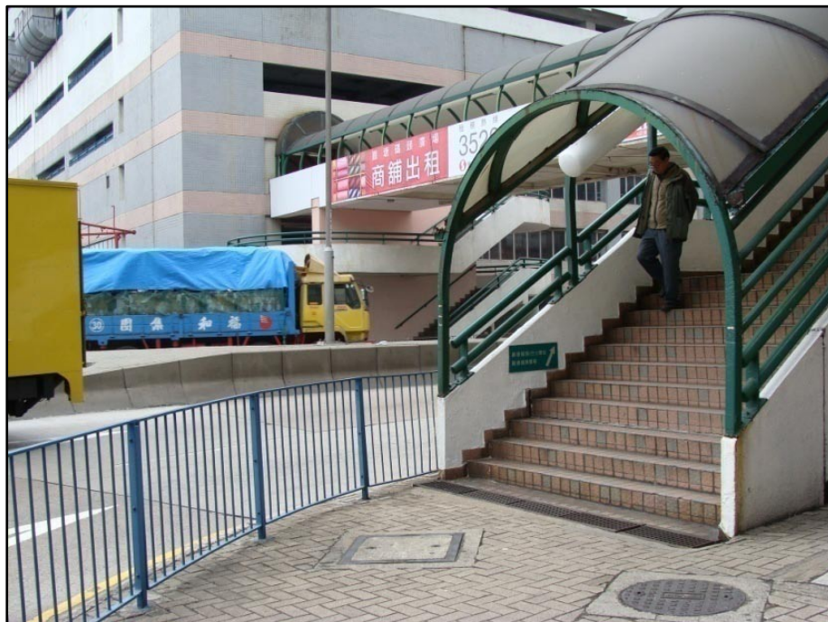
Figure 5.2: Overpass without handicap access in Kwun Tong
