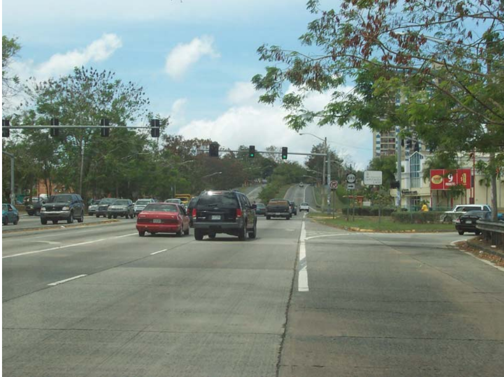
Figure 65: 848 Intersection Looking North
