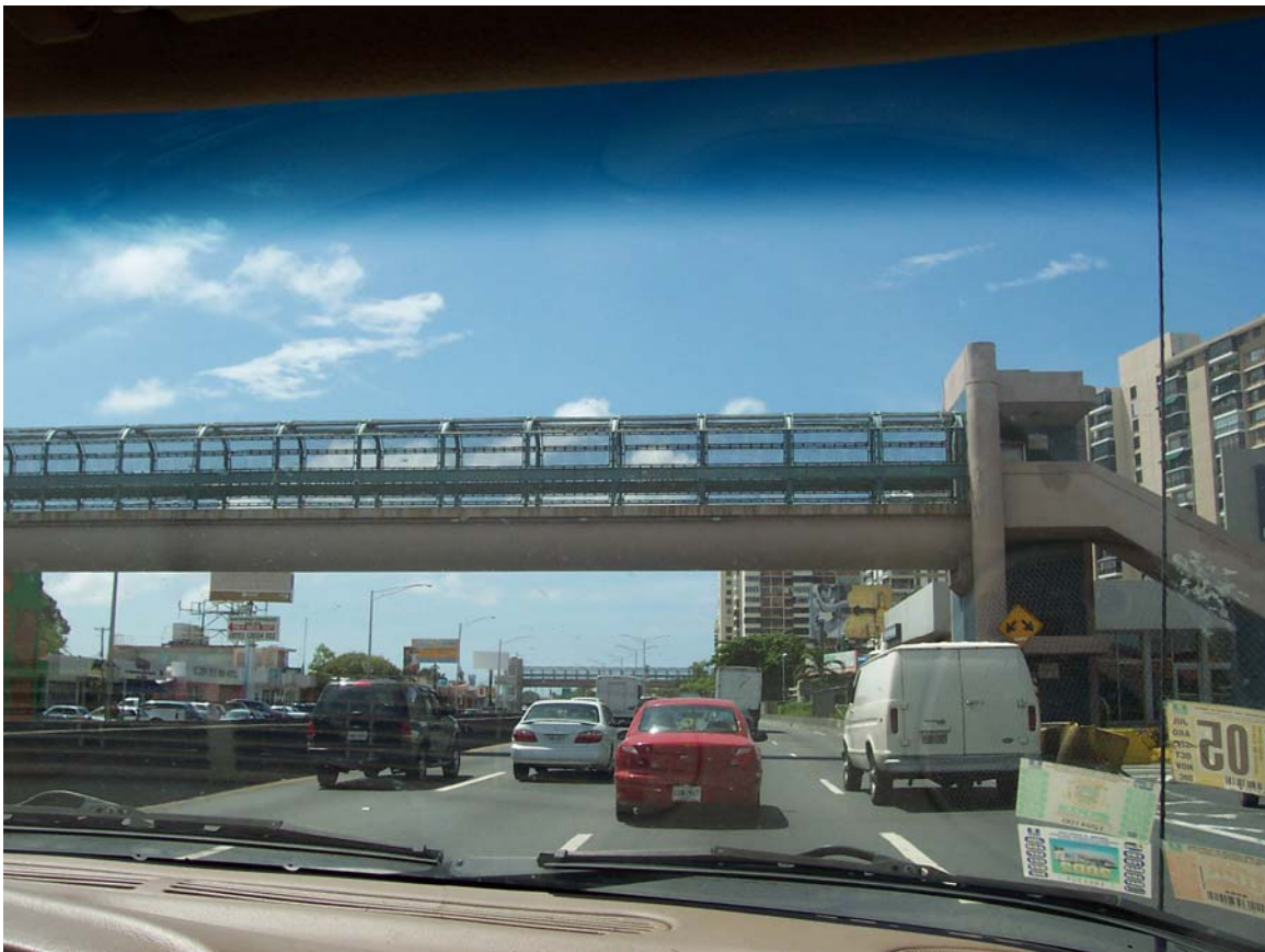
Figure 28: Example of Pedestrian Bridge along PR-26
