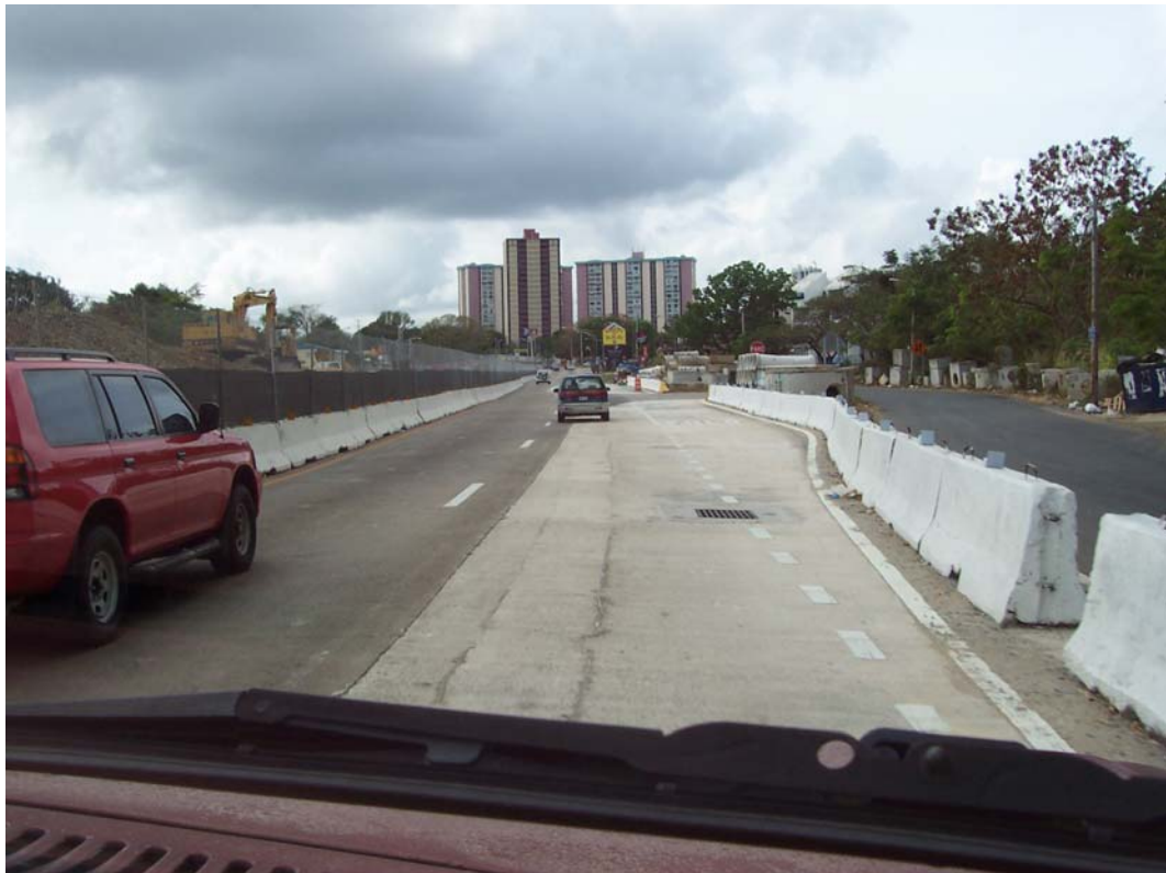
Figure 70: 181 South Heading to Park Gardens Intersection
