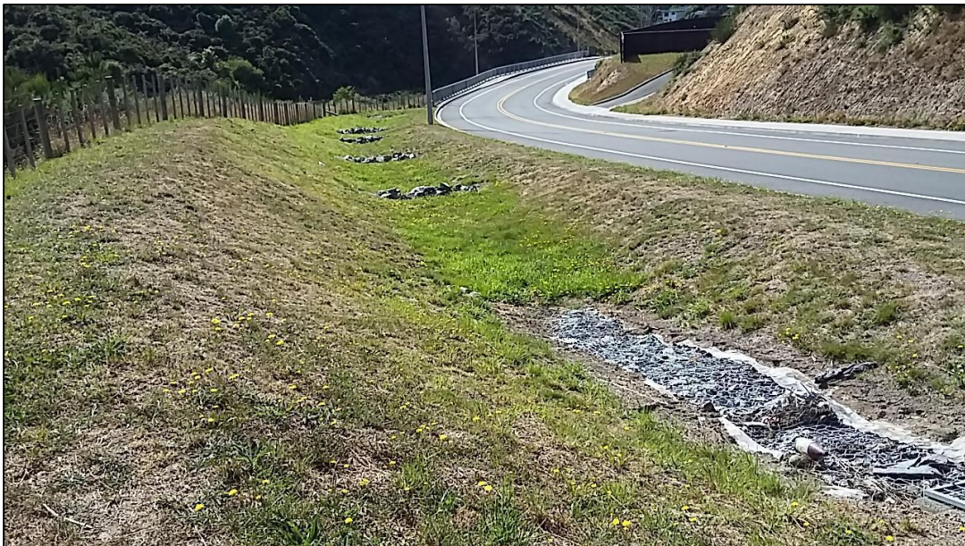
Figure 2: Swale in Porirua
