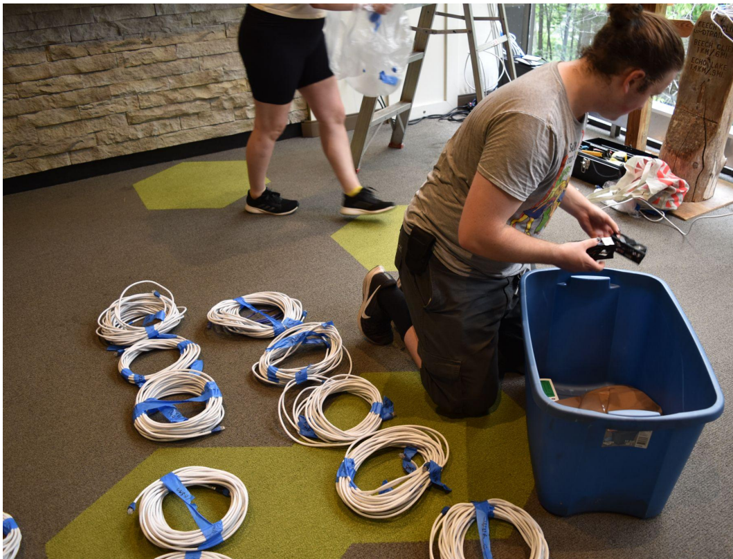
Figure 32: Neatly coiled ethernet cables
