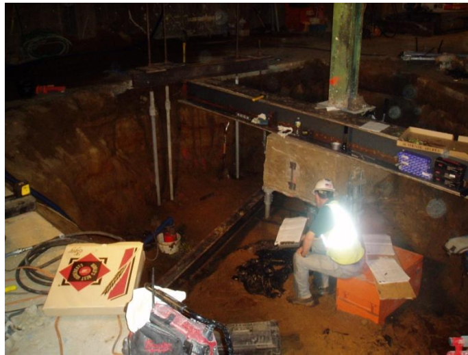
Figure 16: Pile Load Testing at Hillsborough County Court House, Manchester NH
