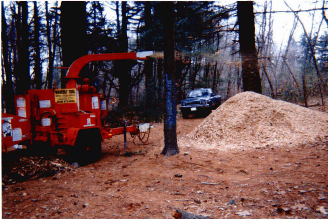
Fig. 14 Wood chipper in service of project
