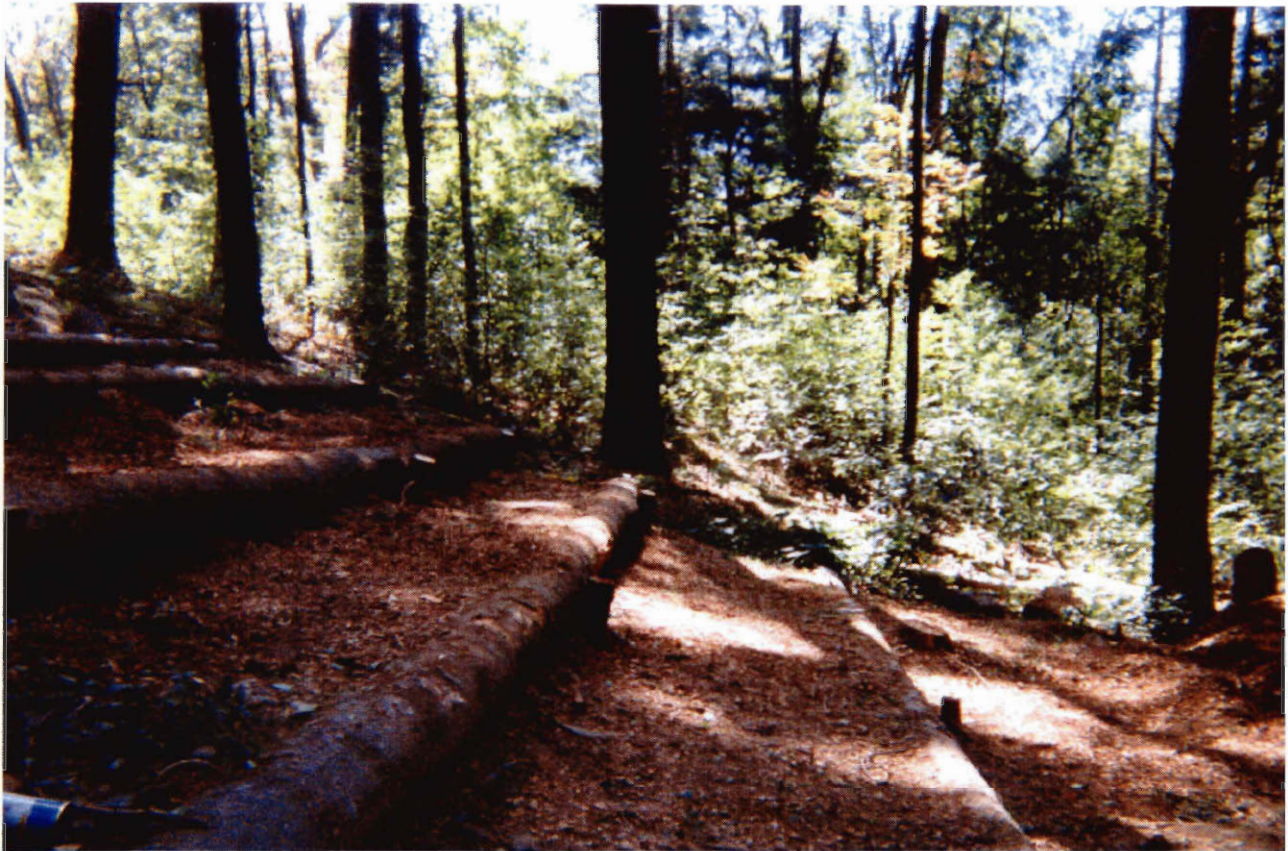
Fig. 22 Side view of completed seating section of amphitheatre
