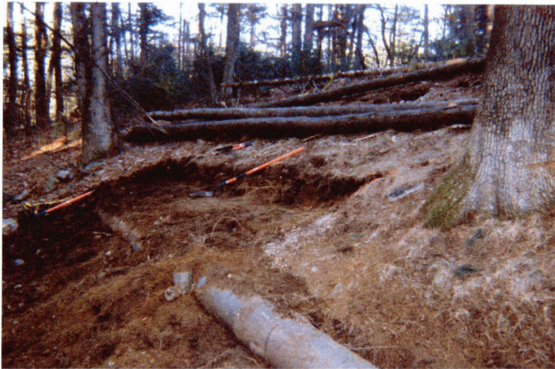
Fig. 17 Excavation to include existing tree
