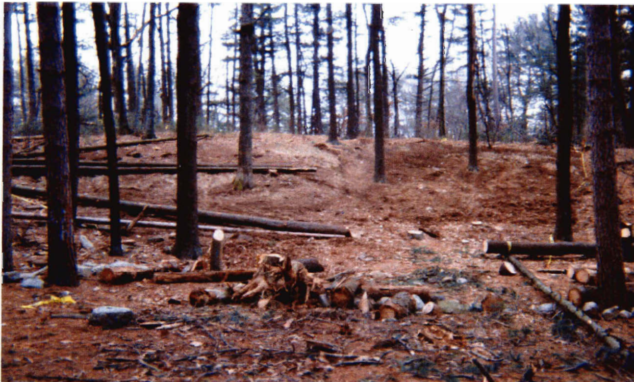
Fig 16 Area cleared for seating construction
