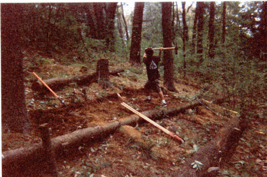
Fig. 18 Fashioning rows by physical work
