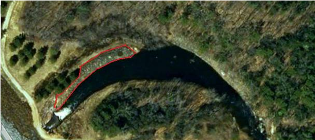
Figure 19: Berm at the East Brimfield Dam (Google Earth 42.109175, -72.126274 2010)
