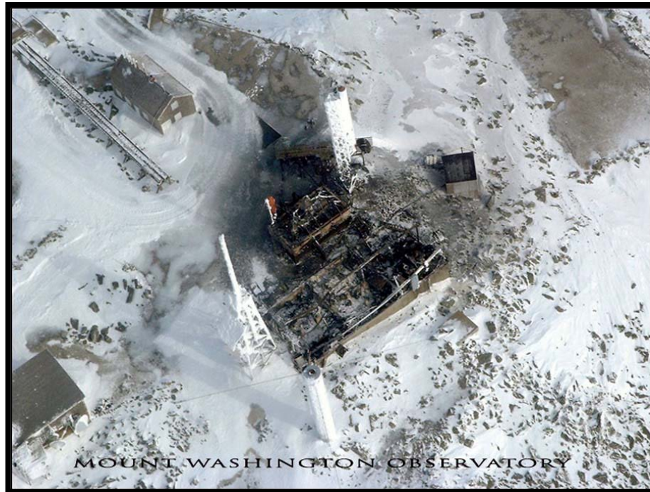
Figure 4: WMTW Building after Fire (Cheshire County DX ARC 2003)
