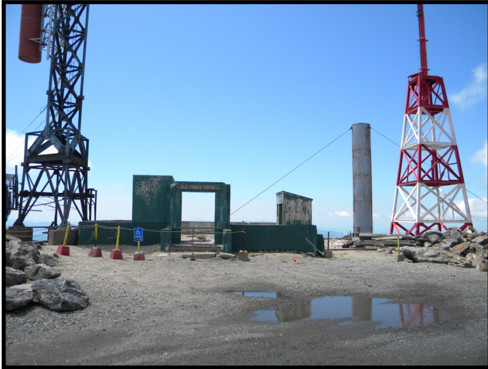
Figure 8: Location of the Old WMTW Building and Proposed Location of the Research Facility
