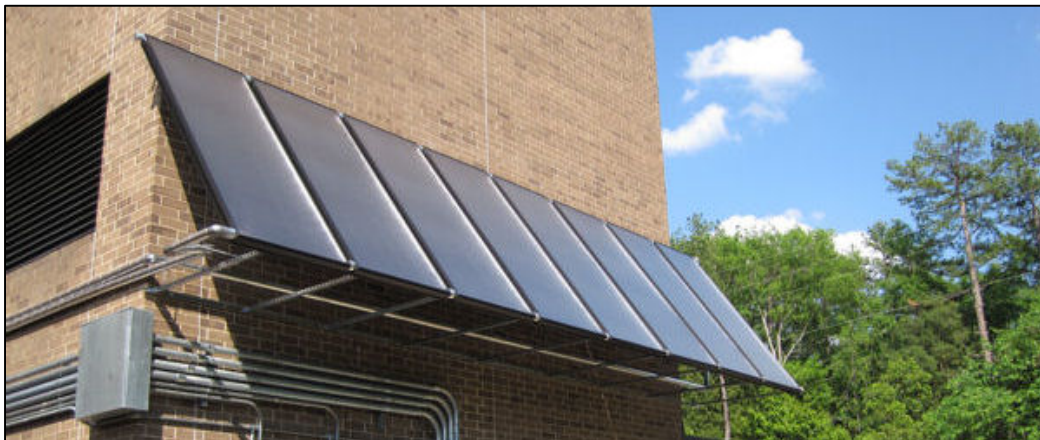
Figure 19 - PV panel wall mounted [23]
