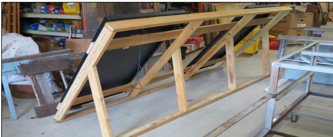
Figure 46 - Custom made ground mounting equipment for the solar panels.
