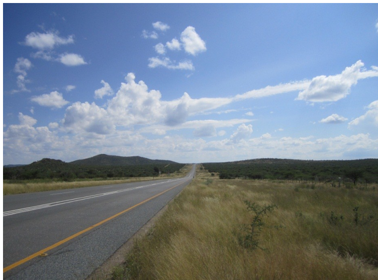
Figure 15: New road surface between Karibib and Okahandja
