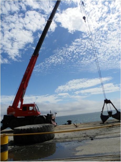
Figure 17: Dredging Crane at Walvis Bay Port
