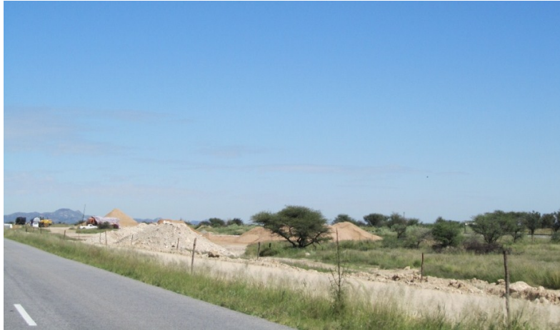
Figure 14: Road construction along the TKC
