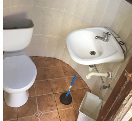
Figure 18: Interior of bathroom facilities at Cabimos (Scammon, 2017)
