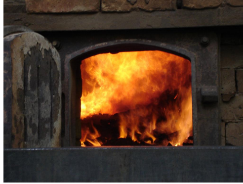
Figure 32: Wood furnace used to burn wood chips (Joseph, 2006)
