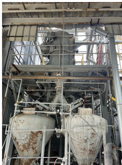
Figure (3) - Silos behind Plant 7
